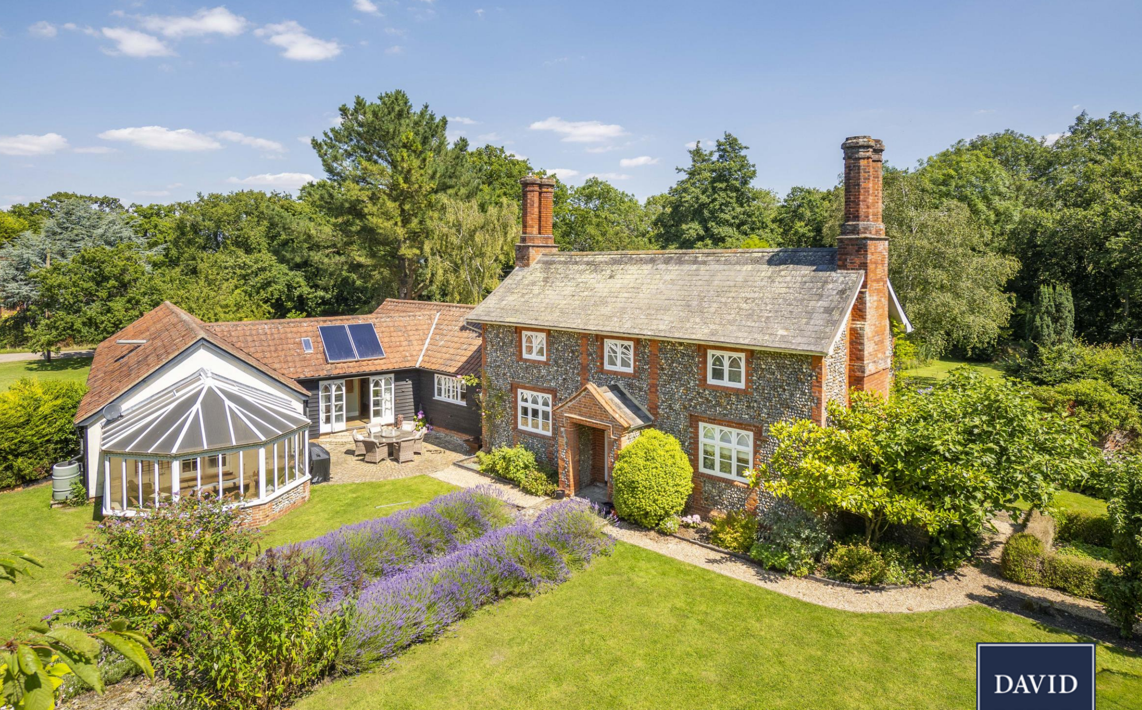
Grove Cottage, Hungry Hall Lane, Long Melford, Suffolk
