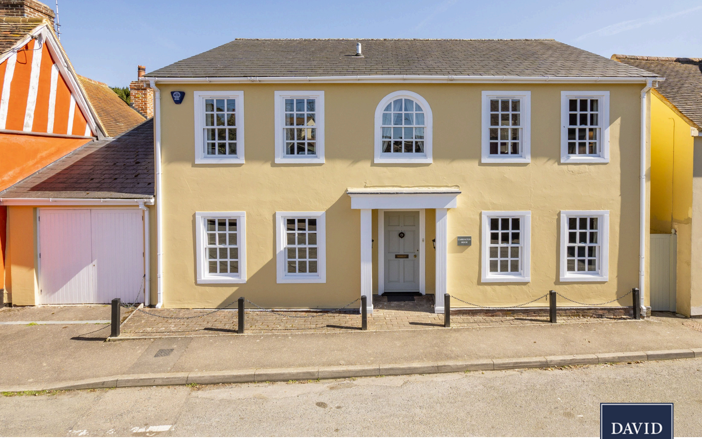
Carrington House, Shilling Street, Lavenham, Suffolk
