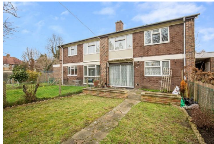
pathway, rear gate access.
