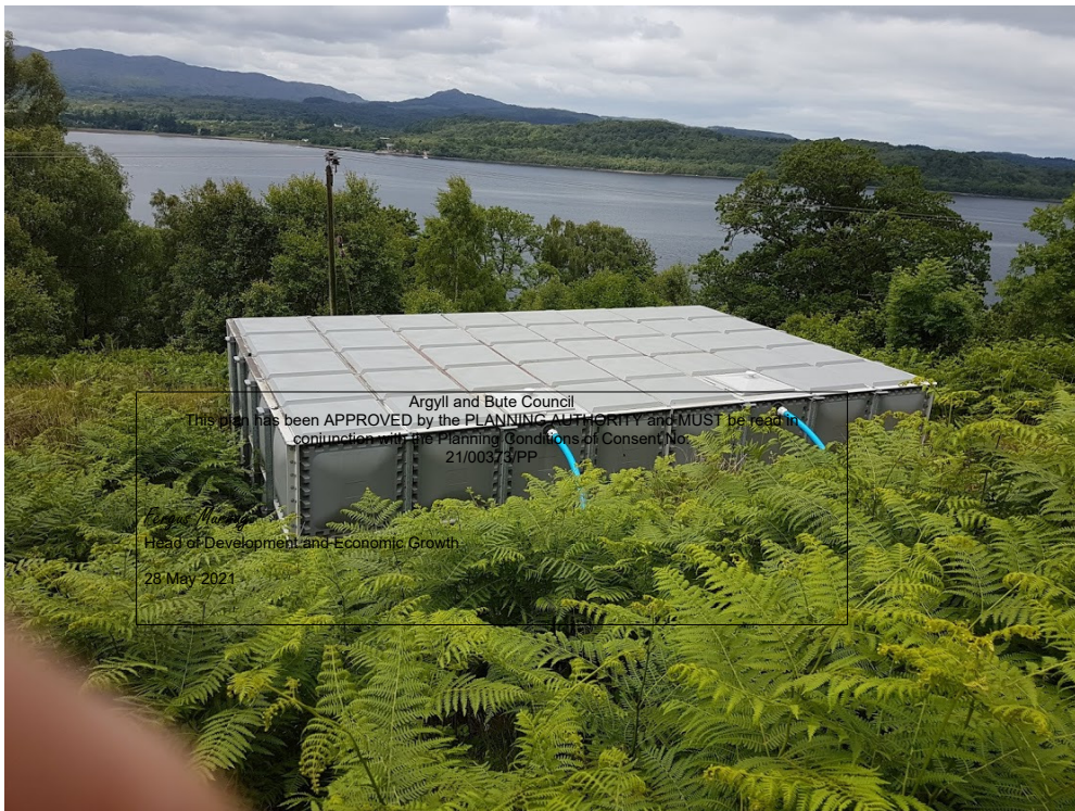
Figure 8 80 cubic metre (80,000 litres) water storage tank
