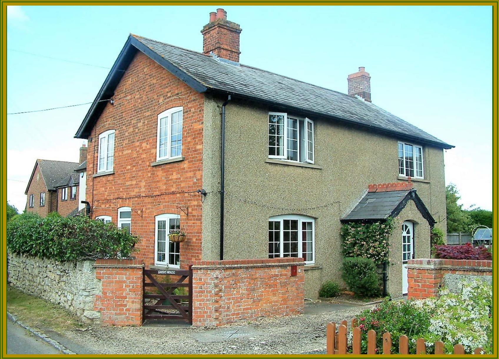
Grove House, Bowling Alley, Oving, Buckinghamshire, HP22 4HD
