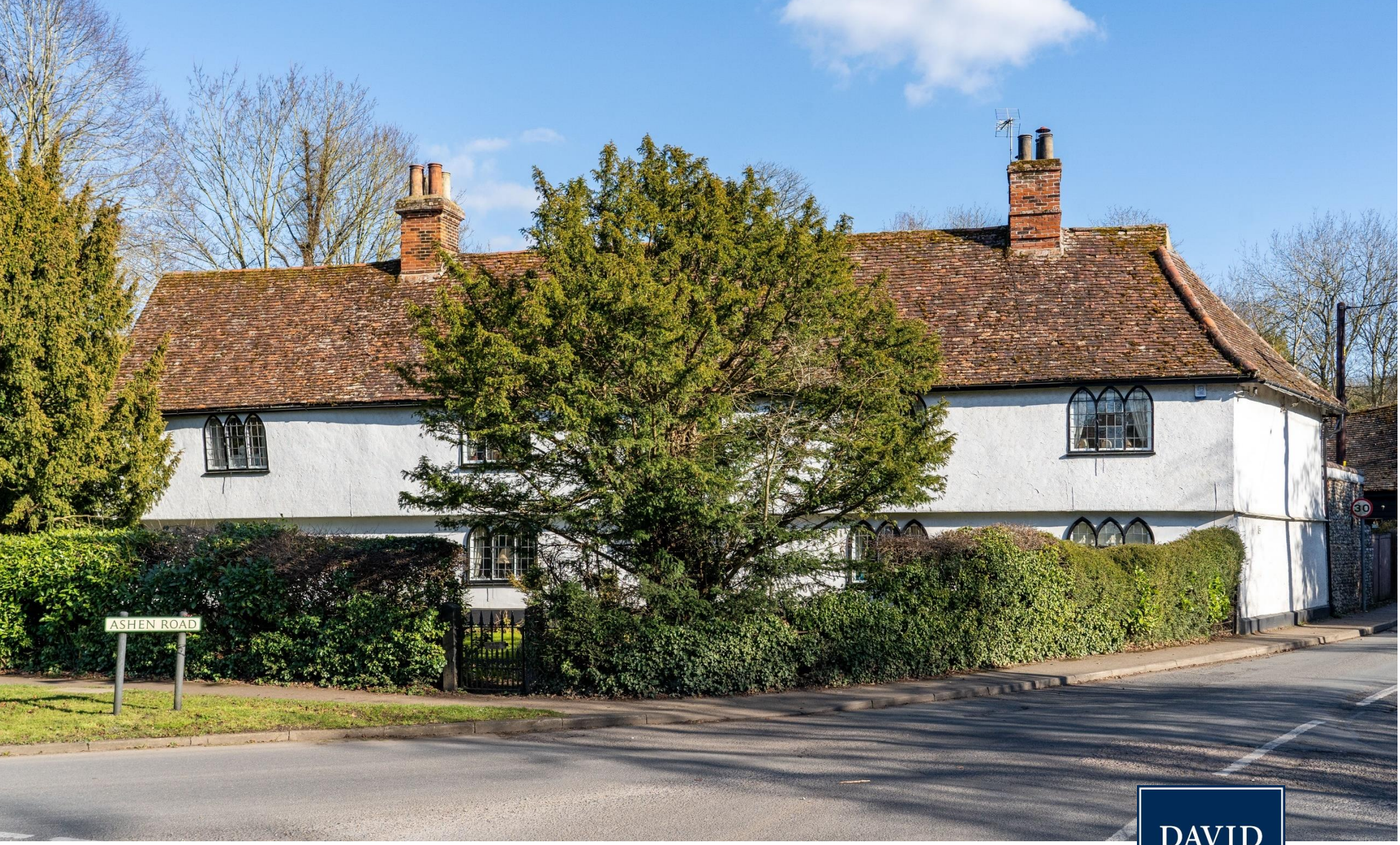
Thornton House Clare, Suffolk
