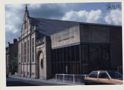
Image credits: Hexham Local History Society. 1971: Gilesgate looking E, No 13 Henry Bell wool warehouse prior to conversion to old swimming pool and demolition of adjoining buildings. 1983: Gilesgate looking N, No 13 Henry Bell wool warehouse/old swimming pool showing swimming pool extension.
