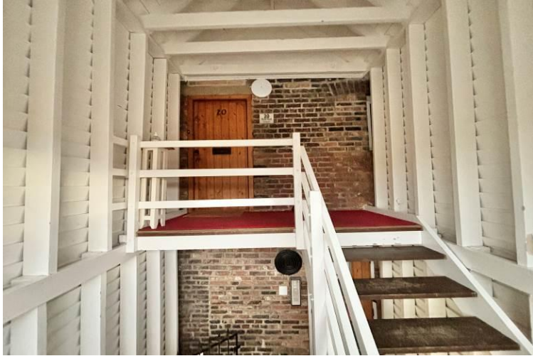
Stairwell to Flat
